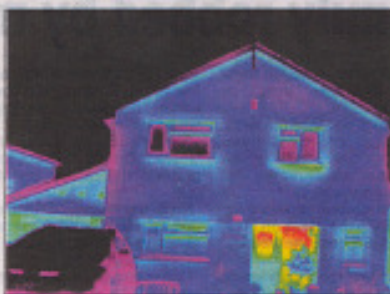
DRIVE-BY INSPECTIONS: The top picture shows a red, poorly insulated home, in contrast to the blue
